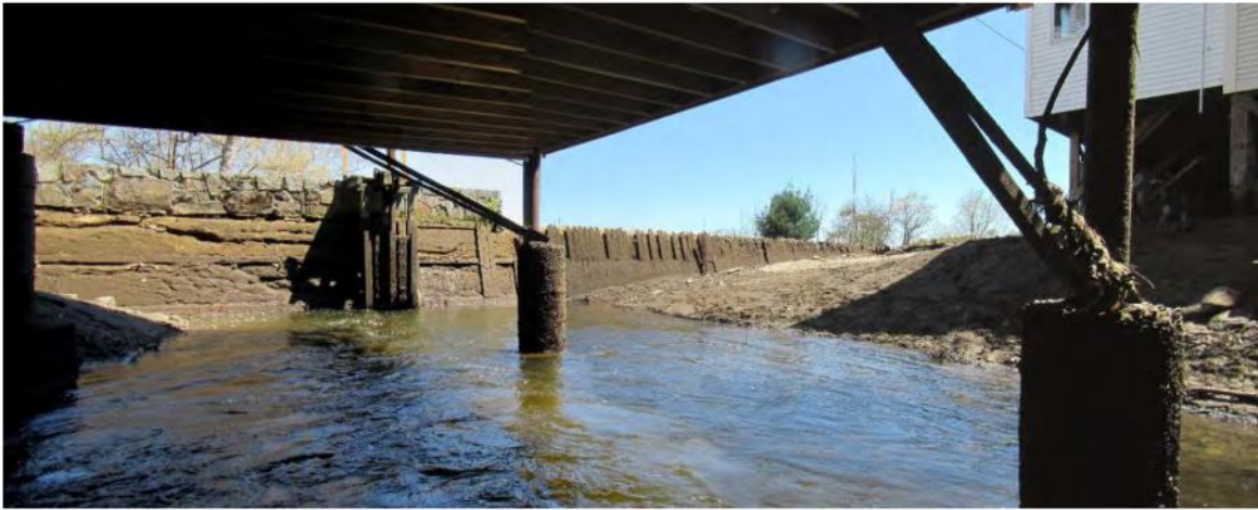
Figure 21. View of lower impoundment in drawn down condition, May 8, 2018. Non-overflow portion of dam and headgate at left half of image, spillway at right half of image. Normal pool elevation at spillway crest.
