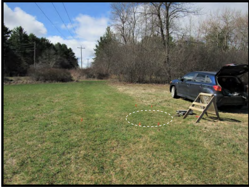
Figure 52: depression and area of excavation (dashed circle) looking south.
