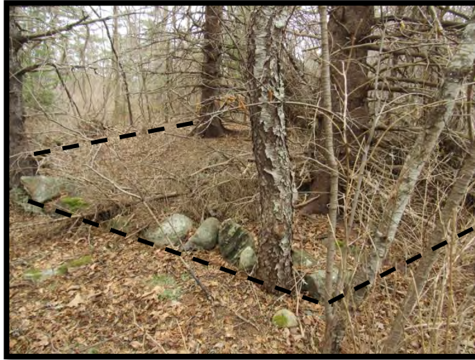
Figure 36: ME 073.014 – barn foundation (facing northeast)
