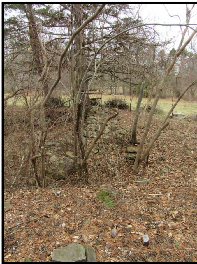
Figure 33: ME 073.014 – cellar (west foundation wall with cellar entrance in foreground)
