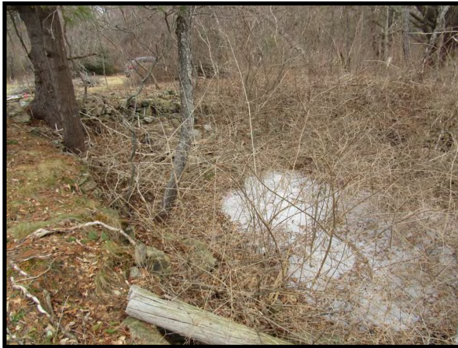
Figure 35: ME 073.014 – south foundation wall looking west northwest
