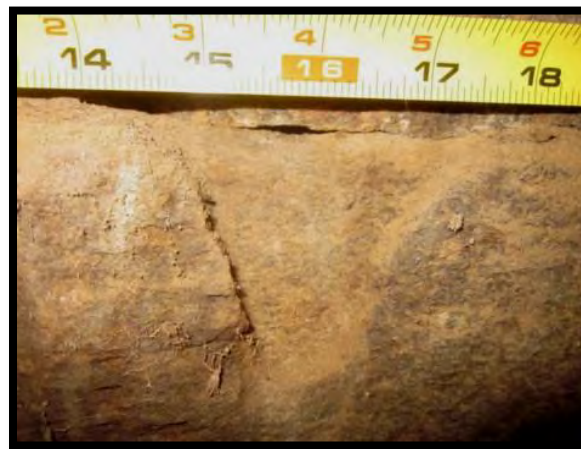
Figure 23: trapezoidal quarry scar indicating use of a cape chisel and flat wedges
