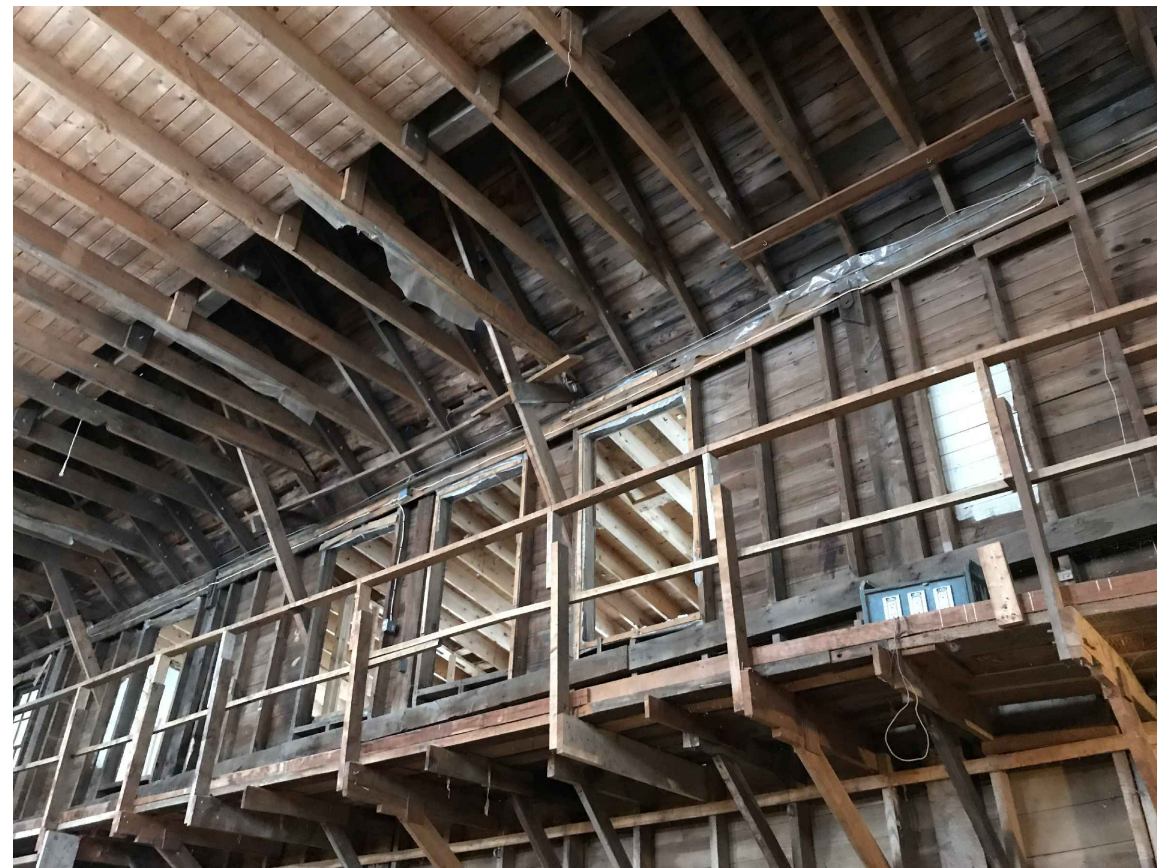
EXISTING ROOF FRAMING AT STORAGE ATTIC
