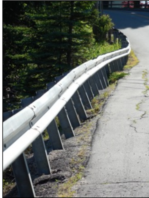
Splayed stanchions can tip a fuel truck or school bus INTO the harbor or lake instead of stopping it (July 2015)
