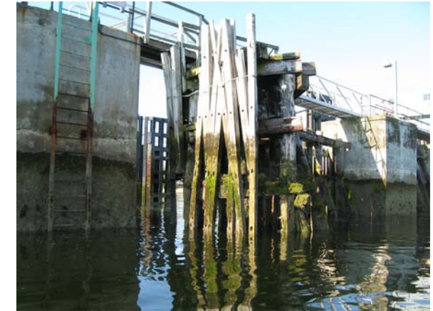
Outer End of Existing Wave Fence
