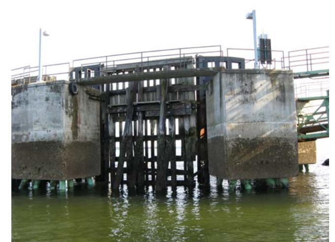
North Side - Existing Inner Section of Wave Fence
