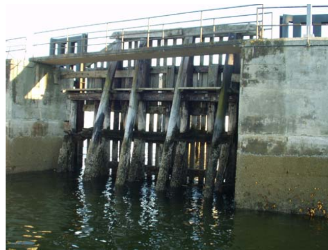
North Side - Existing Middle Section of Wave Fence
