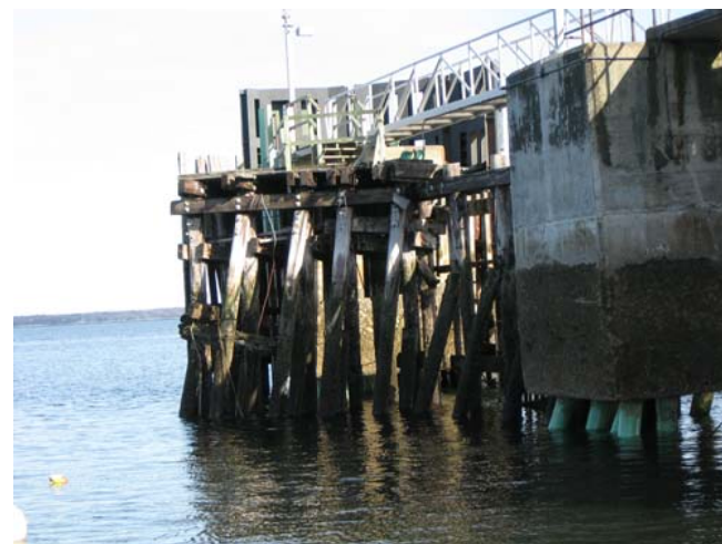
North Side - Existing Outer Section of Wave Fence
